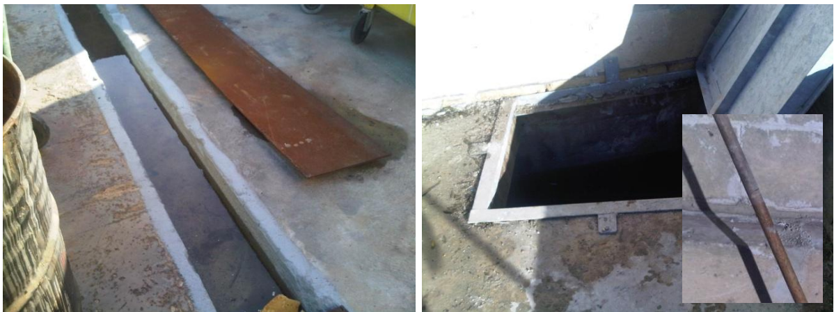
Photo 2: Spill channel and cesspit (with dipstick insert) after 24 hrs
